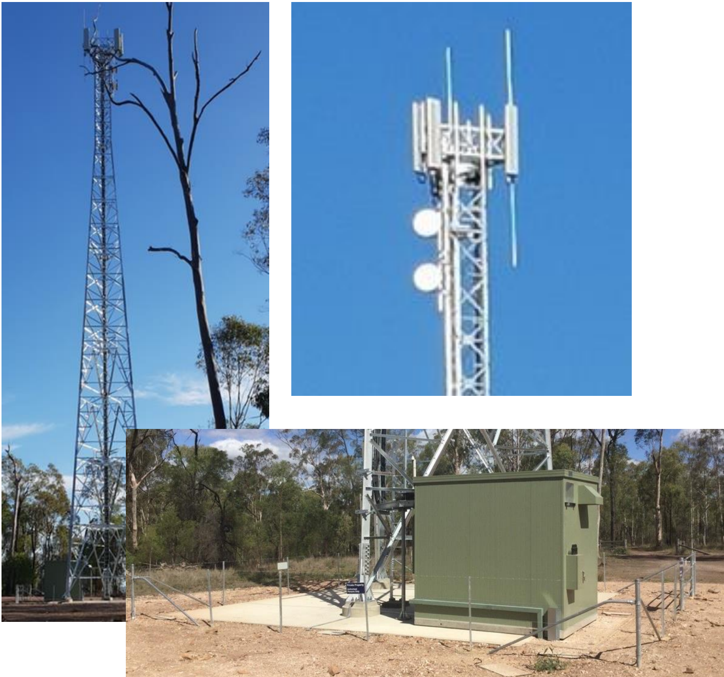
Figure 1: Left: Constructed 60m lattice tower. Top right: Example of proposed headframe design. Bottom right: Lattice tower base including equipment shelter and stock fence Source: Visionstream 2019
