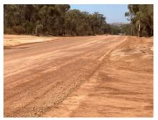
The construction phase of stage two of the Wickepin-Pingelly Road and Old Wickepin Road intersection is now complete. Testing is now being undertaken prior to sealing. The stage three works are currently being marked out in preparation of the commencement of works.
